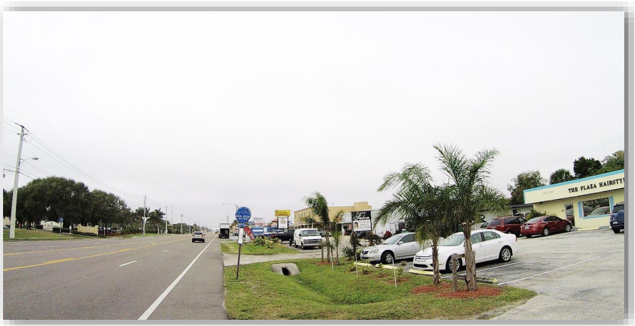
Exhibit 2 – Bus Stop with No Amenities
