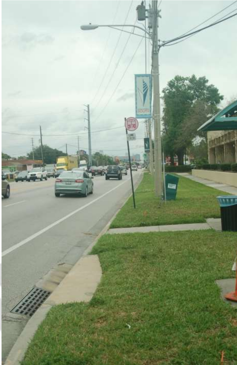
Figure 22: Sidewalk Setback on Orange Avenue between Pineloch Avenue and Michigan Street.
