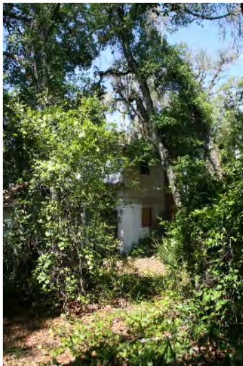
8VO09385_c Facing Southwest
