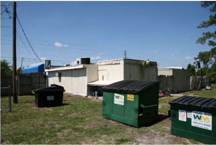
8VO09384_c Facing Southwest
