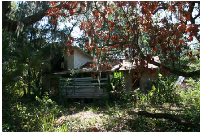
8VO09385_d Facing East
