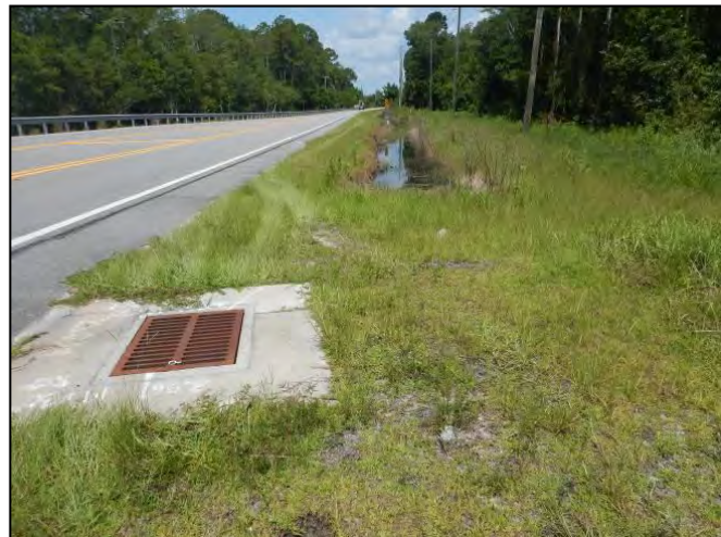
Figure 15. Overview of west end of Pioneer Road, north side, view west.
