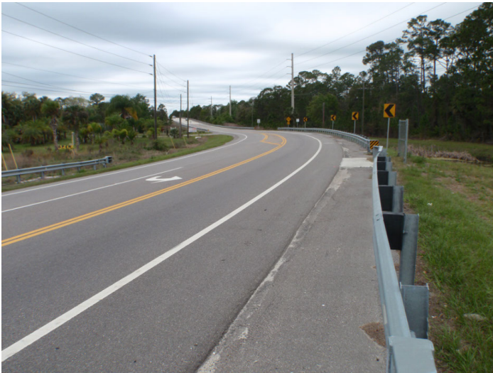
8VO07656_c Facing West
