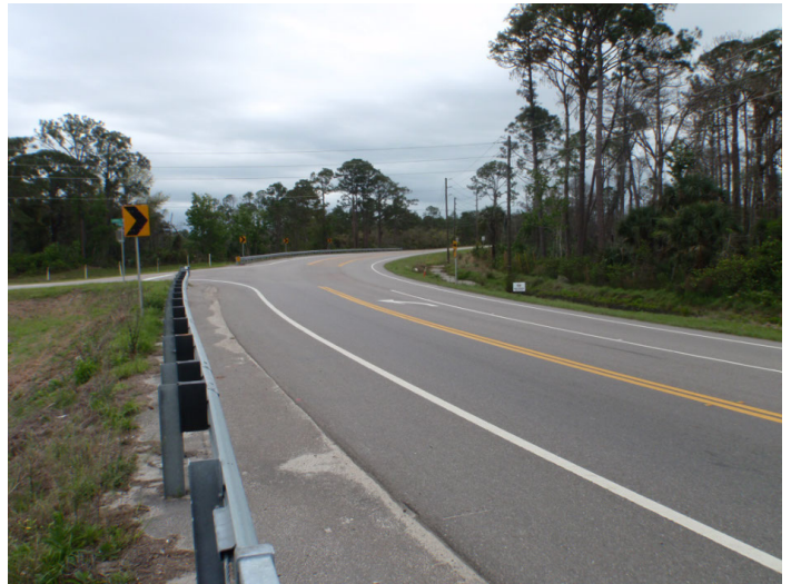
8VO07660_d Facing East
