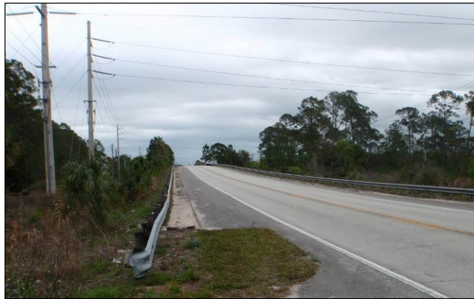
Figure 16. Resource 8VO07660, facing east and showing above-ground disturbances.
